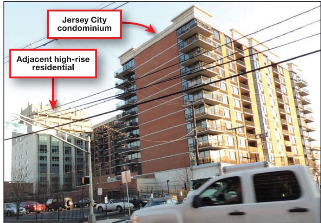
Figure 4-13: A Jersey City condominium and adjacent interconne building (Jersey City, NJ)
