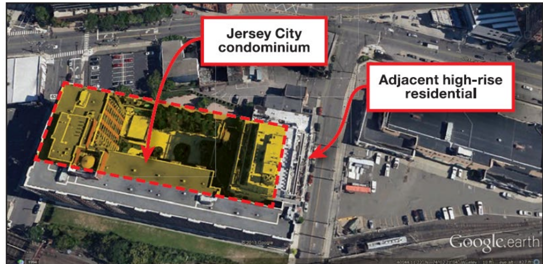
Figure 4-14: Aerial view of a Jersey City condominium and adjacent building where highlighted region show approximate location of two-level parking garag located partially beneath both buildings (Jersey C NJ)
